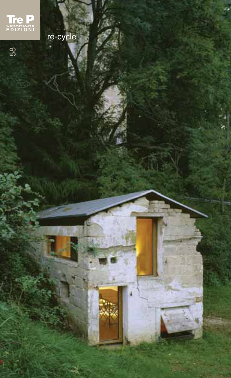
S(ch)austallnaumann. architektur Ramsen, Germania / Germany 2004 - 2005 ante e post intervento
